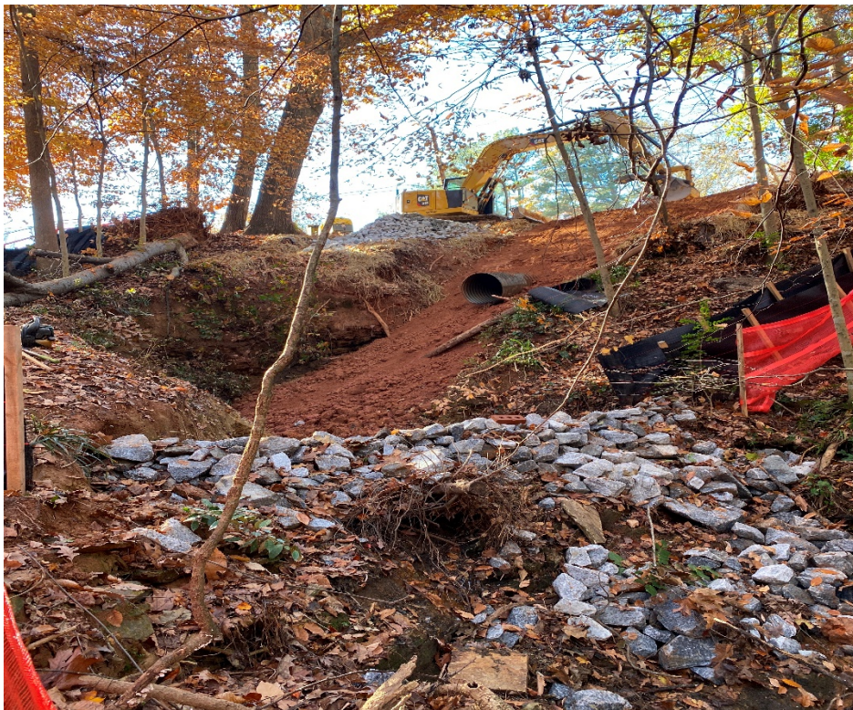
New Drainage pipe installed.
