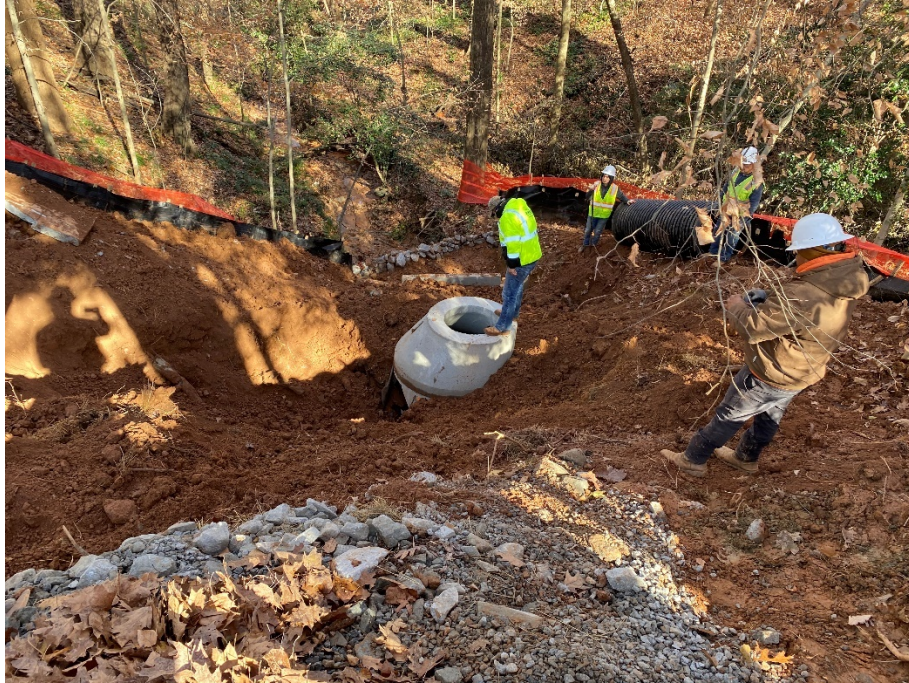
Installing the drainage Pipe.
