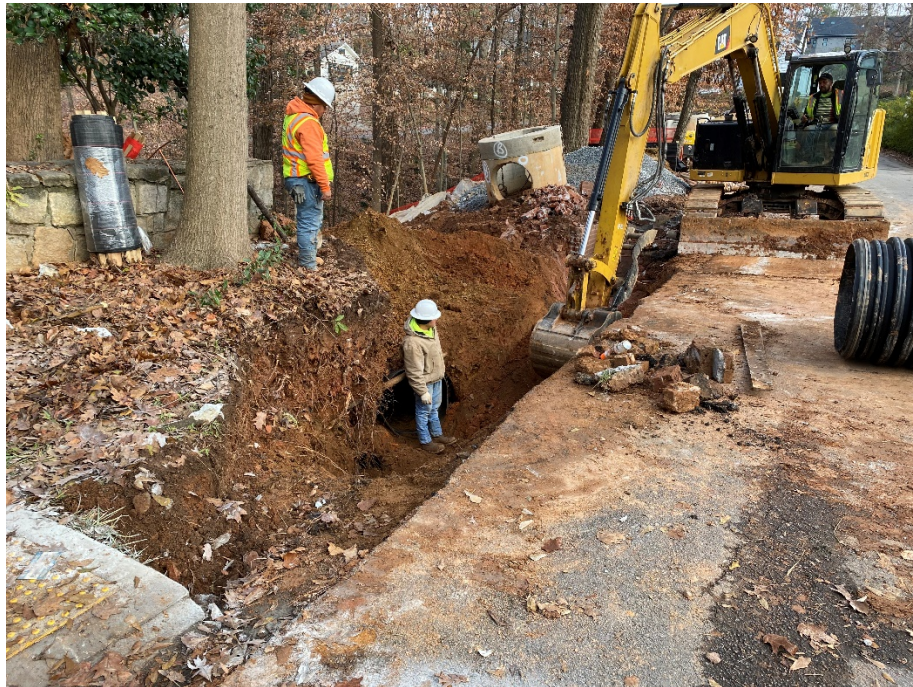
Installing the drainage Pipe.
