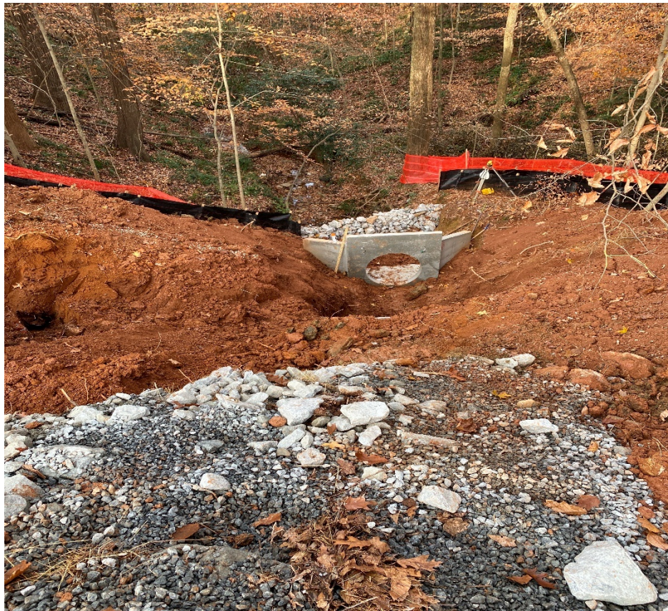
Headwall being installed.
