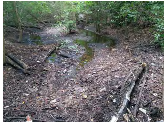
Figure 2-23. Example of a Non-Functional Stormwater Management Structure Needing Maintenance
