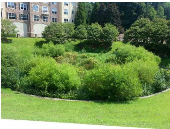
Figure 2-22. Example of a Functional and Well-Maintained Stormwater Management Structure
