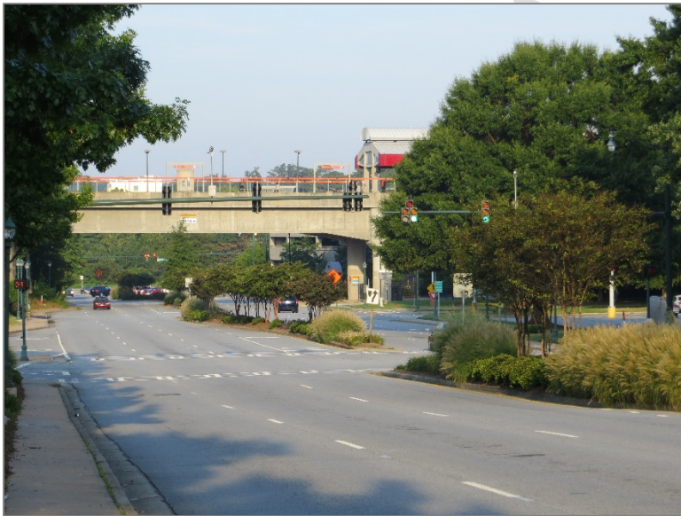
FIGURE 3. VIEW OF DUNWOODY MARTA STATION SEEN FROM HAMMOND DR
