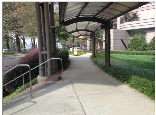
FIGURE 1. COVERED WALKWAY BETWEEN SANDY SPRINGS MARTA STATION AND NORTHPARK OFFICE COMPLEX
