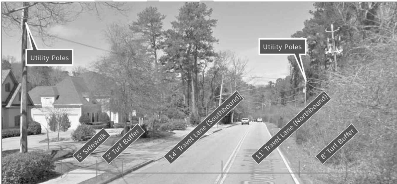
FIGURE 4. EXISTING ROAD CONFIGURATION IN SEGMENT 1 (FACING NORTH).
