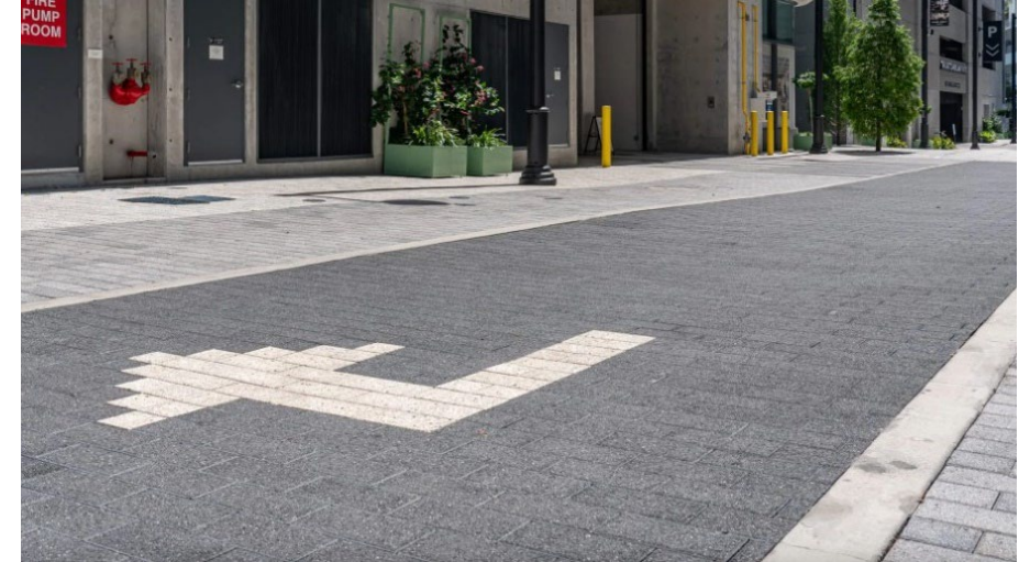
VEHICULAR PAVERS AT WEST PLAZA DEDUCT ALTERNATE: INTEGRALLY COLORED CONCRETE PAVEMENT WITH ACID WASH FINISH
