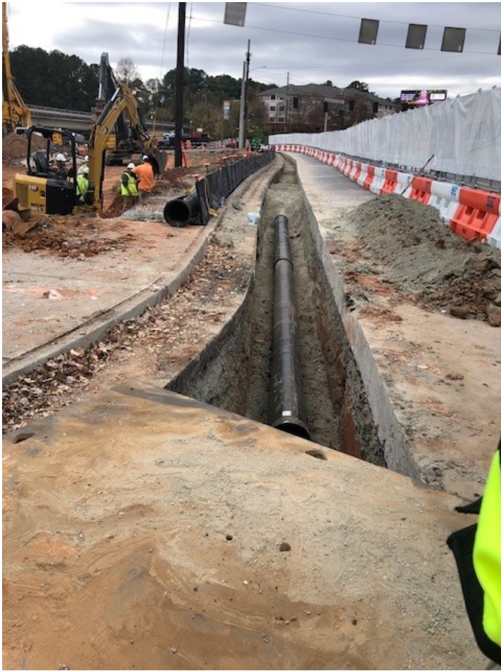
New Water line
