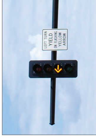
Flashing Yellow Arrow (FYA)
