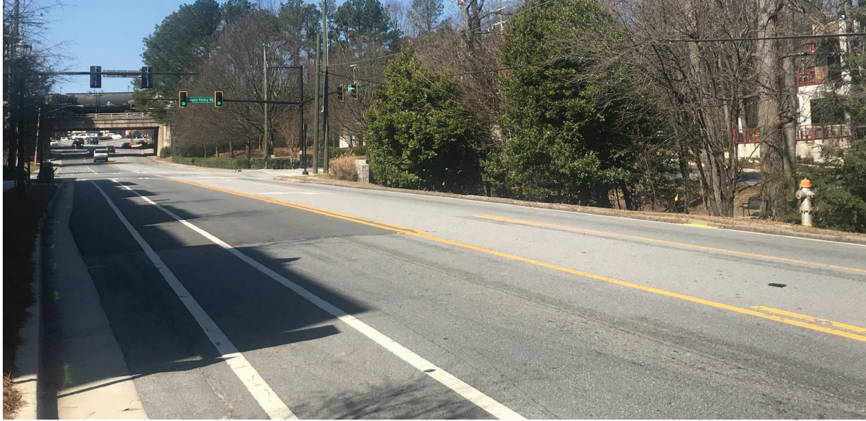
FIGURE 9: WIDE SHOULDER ALONG DRESDEN DRIVE EAST OF APPLE VALLEY ROAD
