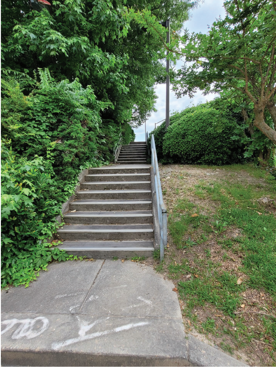
STAIRCASE LEADING TO BROOKHAVEN-OGLETHORPE MARTA STATION FROM THE SOUTHWEST CORNER OF THE INTERSECTION
