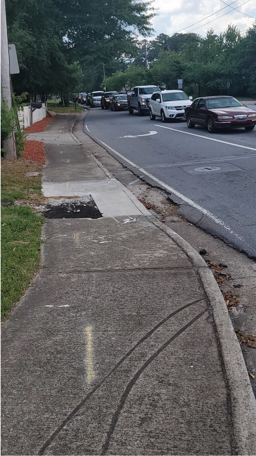
TRAFFIC QUEUING ON EASTBOUND DRESDEN DRIVE AND DEAD-END SIDEWALK ON THE SOUTH SIDE OF DRESDEN DRIVE
