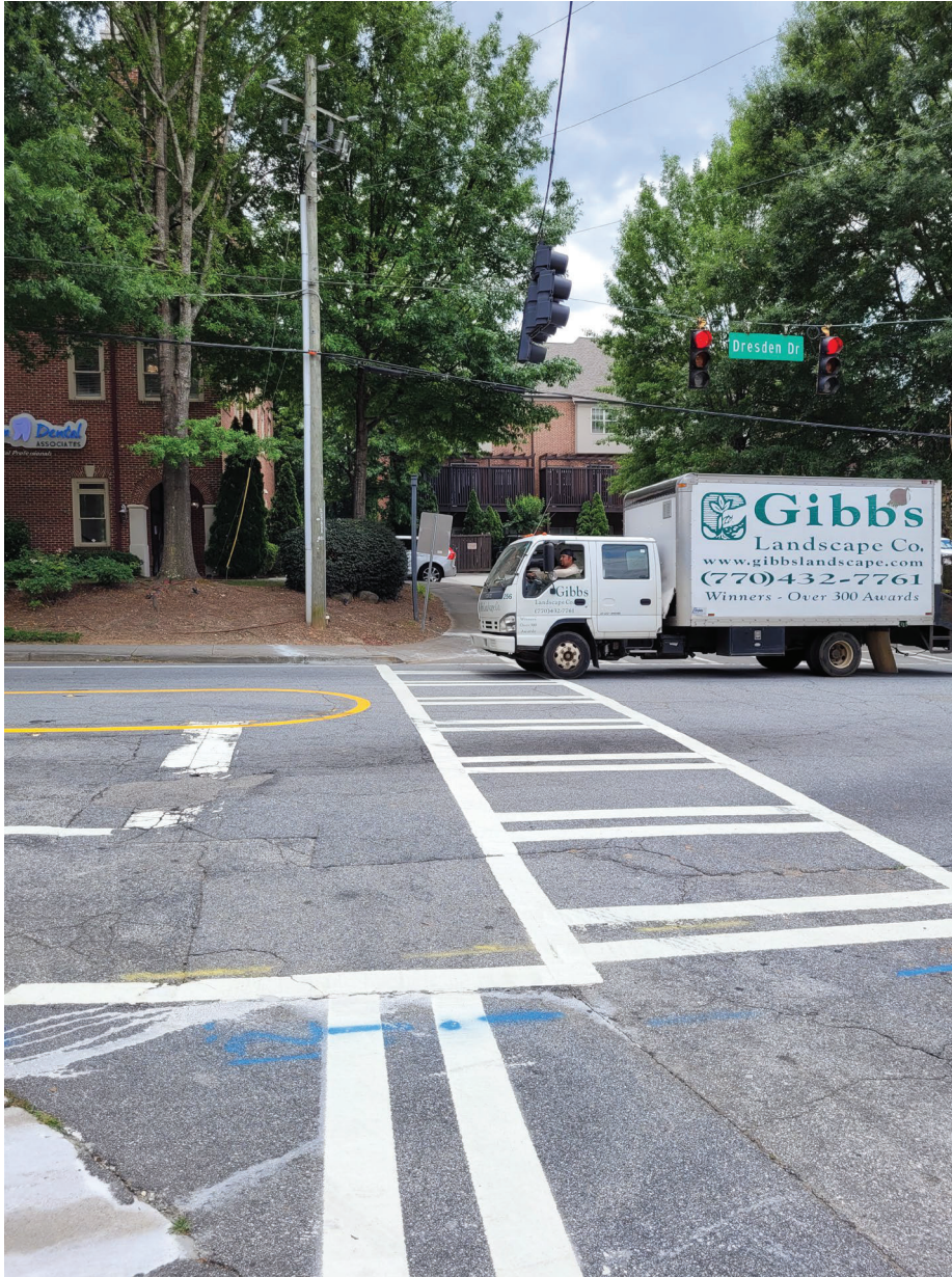
CROSSWALK MARKINGS IN THE EAST LEG IN GOOD CONDITION, BUT NO PEDESTRIAN CROSSING SIGNAL PRESENT
