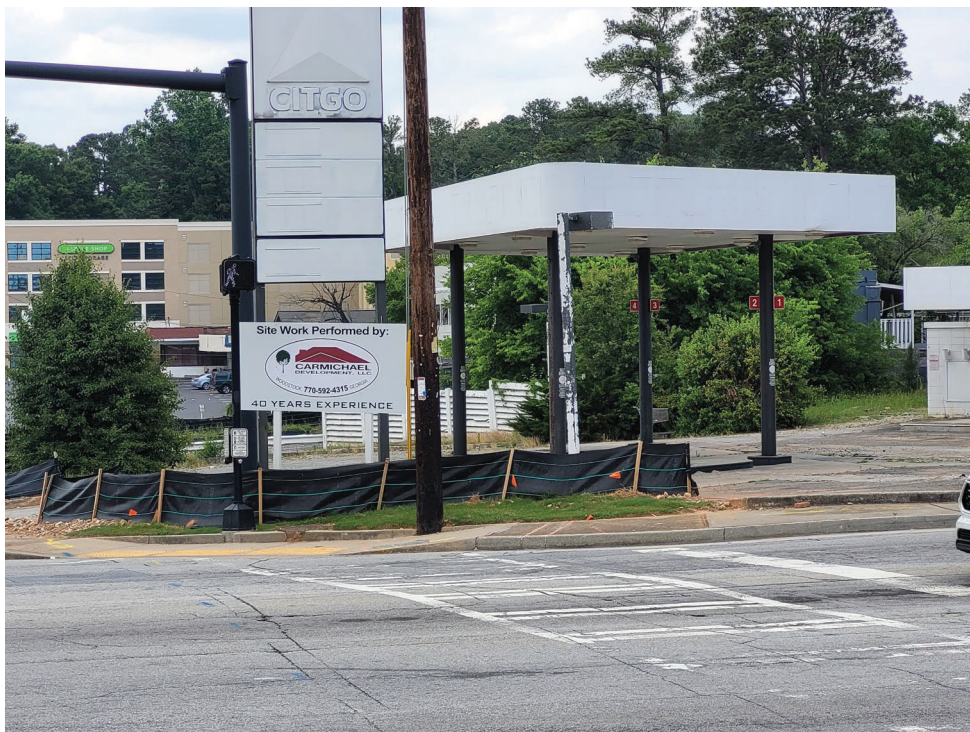
SITE DEVELOPMENT WORK UNDERWAY AT FORMER GAS STATION ON THE NORTHEAST CORNER OF THE INTERSECTION
