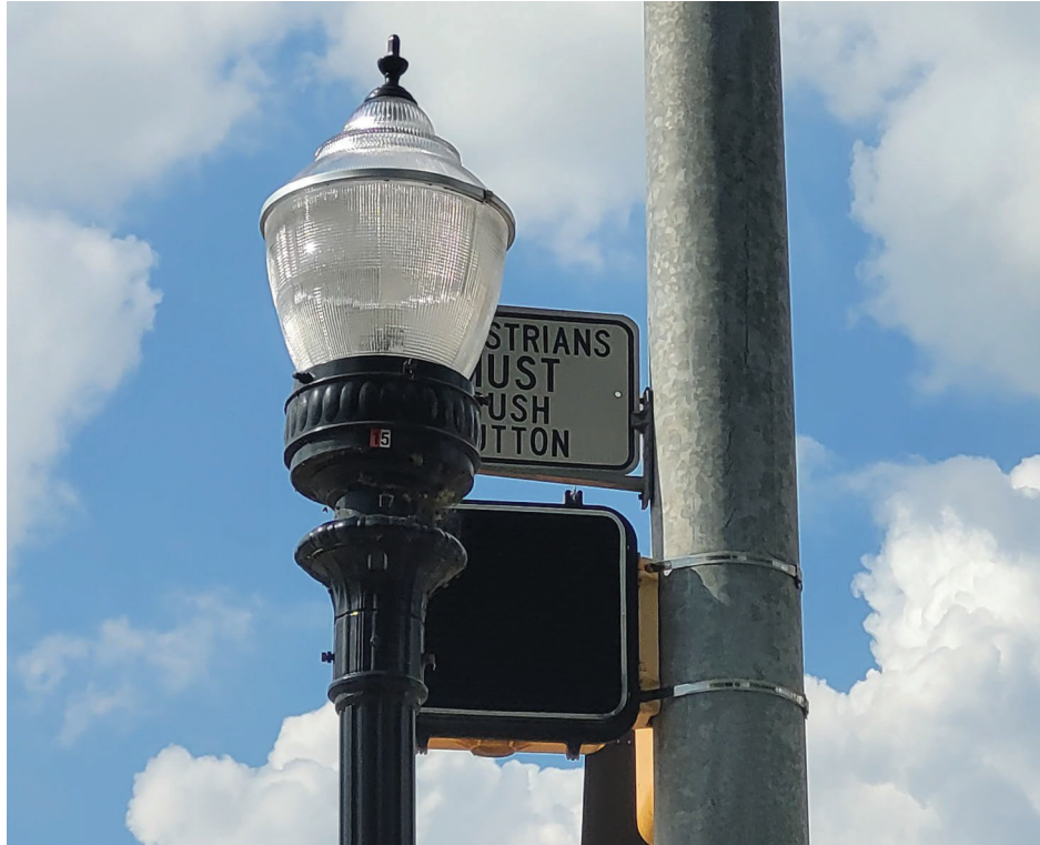
CROSSING SIGNAL PLACEMENT TOO HIGH AND BEHIND THE LAMPOST IN THE NORTHWEST CORNER OF THE INTERSECTION
