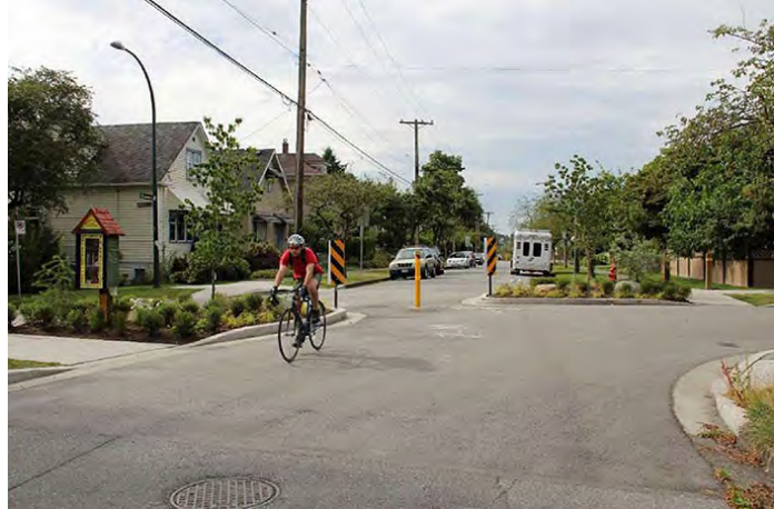
FIGURE 23: EXAMPLE OF A DIAGONAL DIVERTER
