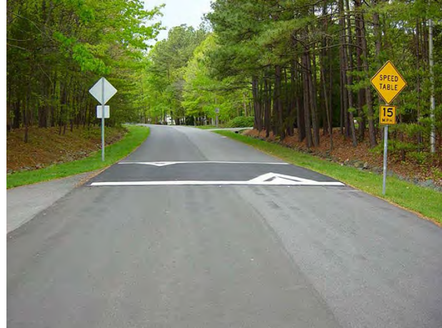
FIGURE 25: EXAMPLE OF A SPEED TABLE
