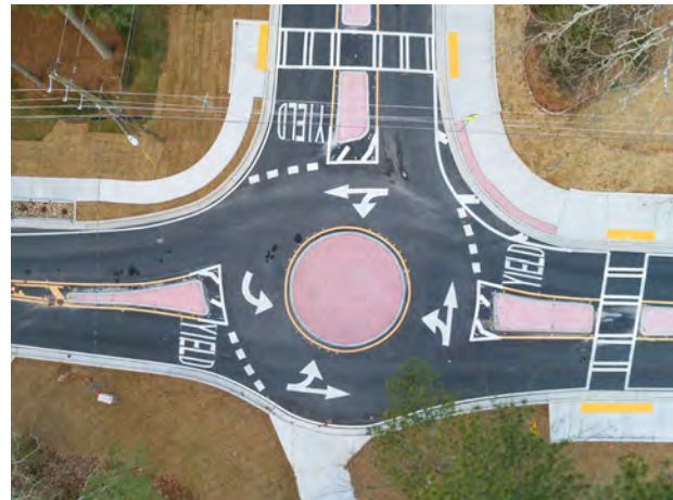
FIGURE 24: EXAMPLE OF A MINI-ROUNDBABOUT
