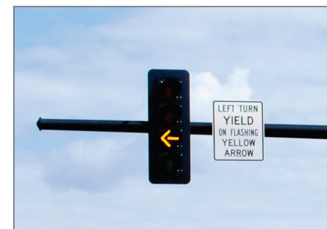
Flashing Yellow Arrow (FYA)
