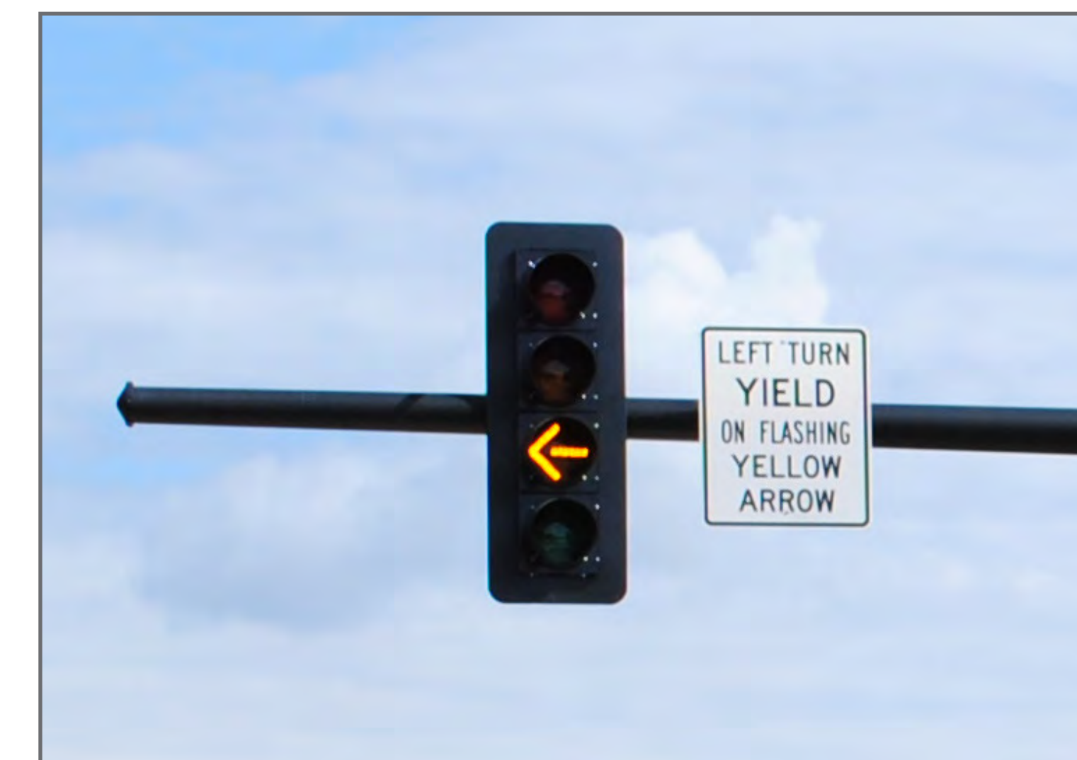
Flashing Yellow Arrow (FYA)
