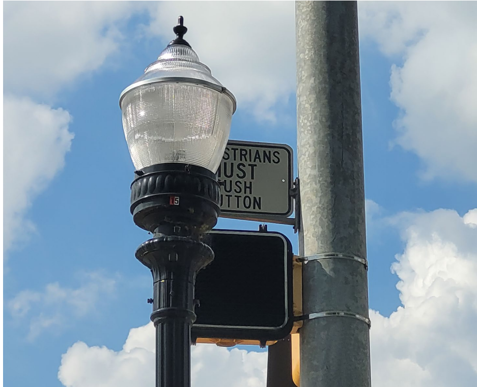
CROSSING SIGNAL PLACEMENT TOO HIGH AND BEHIND THE LAMPOST IN THE NORTHWEST CORNER OF THE INTERSECTION
