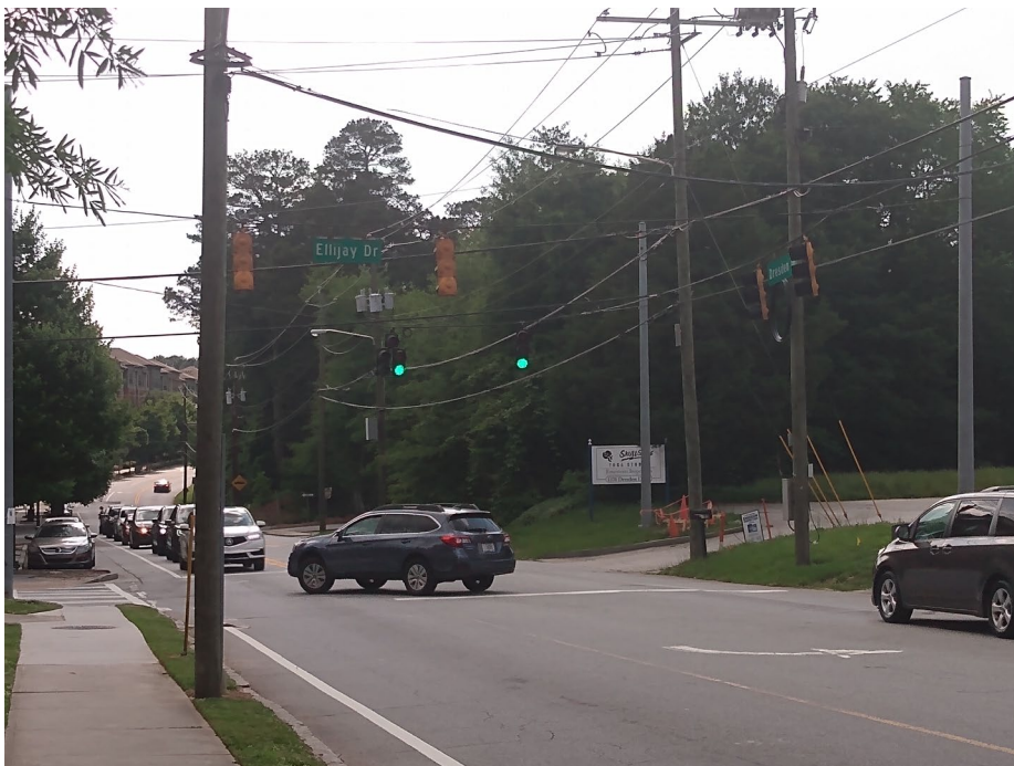
GREEN ARROW DOES NOT TURN ON AT THE ELLIJAY DRIVE INTERSECTION FOR VEHICLES IN THE LEFT-TURN LANE
