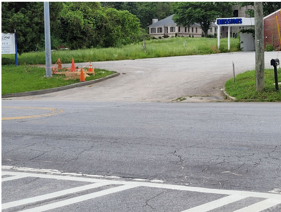
NO SIDEWALK OR CURB RAMPS ON THE NORTH SIDE OF DRESDEN DRIVE BETWEEN PARKSIDE DRIVE AND CALDWELL ROAD
