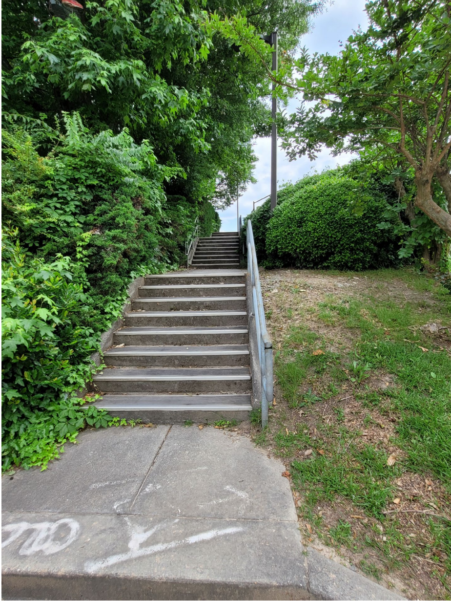
STAIRCASE LEADING TO BROOKHAVEN-OGLETHORPE MARTA STATION FROM THE SOUTHWEST CORNER OF THE INTERSECTION
