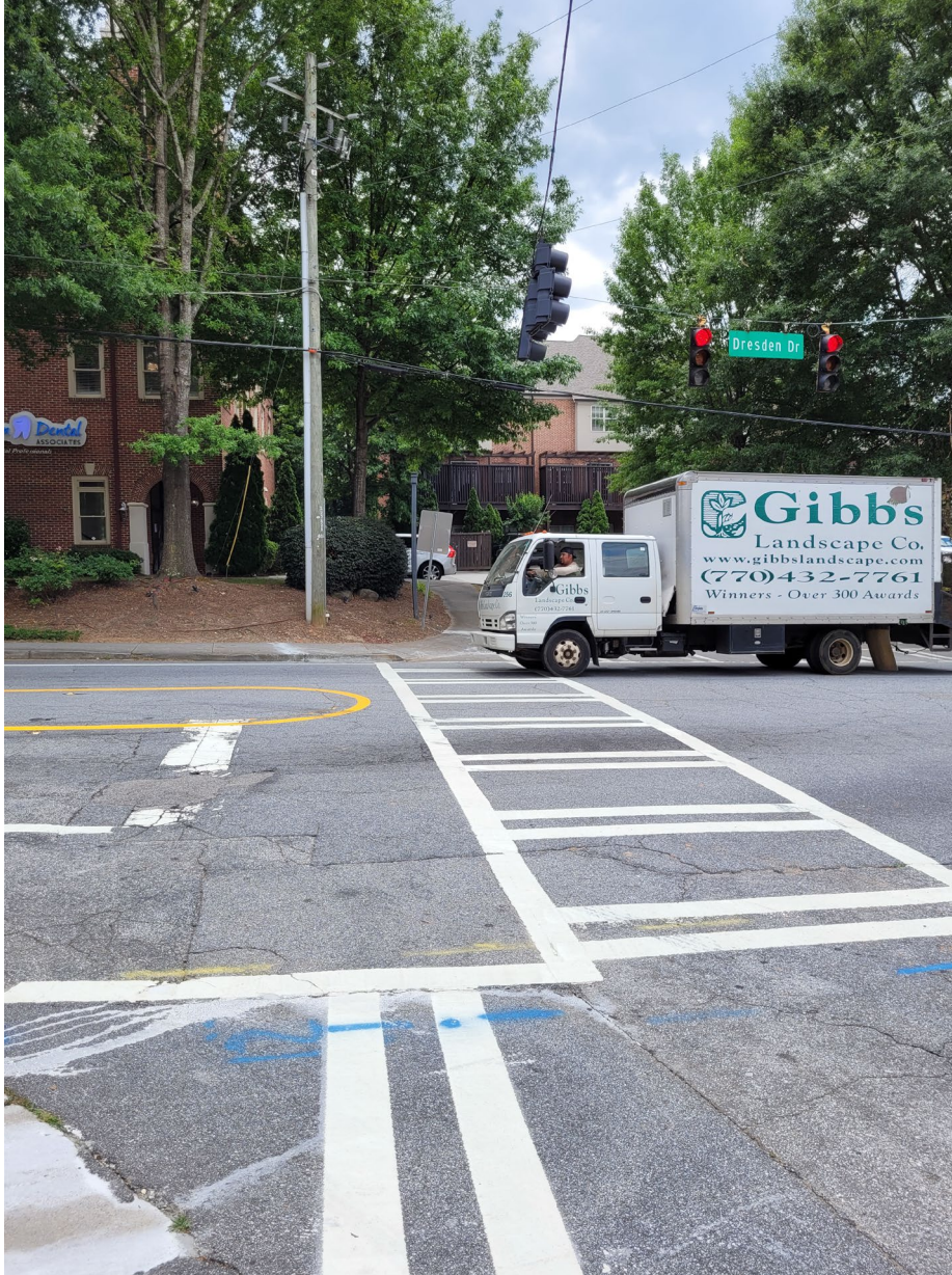
CROSSWALK MARKINGS IN THE EAST LEG IN GOOD CONDITION, BUT NO PEDESTRIAN CROSSING SIGNAL PRESENT
