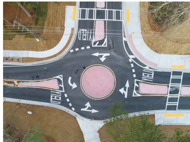
FIGURE 24: EXAMPLE OF A MINI-ROUNDBABOUT
