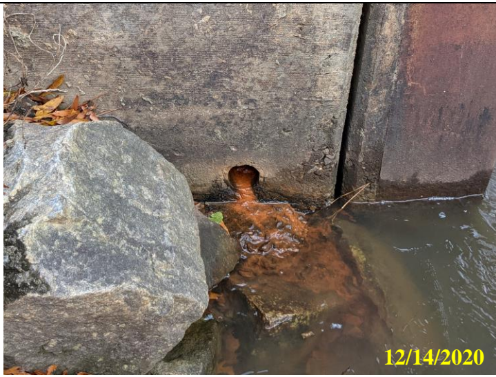
25. Toe drain at right side of plunge pool discharging rust colored liquid
