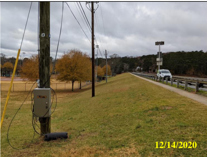
17. View of downstream slope looking toward right abutment
