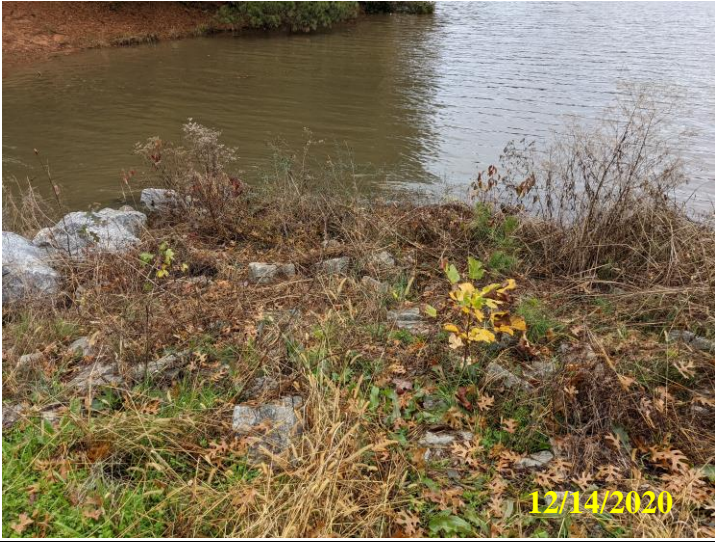
9. View of vegetation on upstream face of the dam
