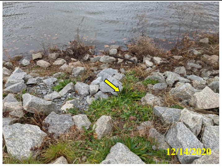
16. Pedestrian pathways showing sparse riprap near principal spillway riser
