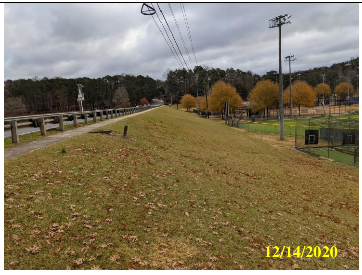
18. View of downstream slope looking toward left abutment
