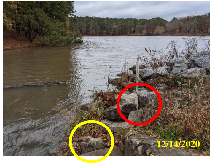
12. Inadequate riprap grading at the left wing wall of the concrete spillway resulting in erosion and undercutting of riprap, yellow circled area is location of Photo 11 and red circled area is location of 13
