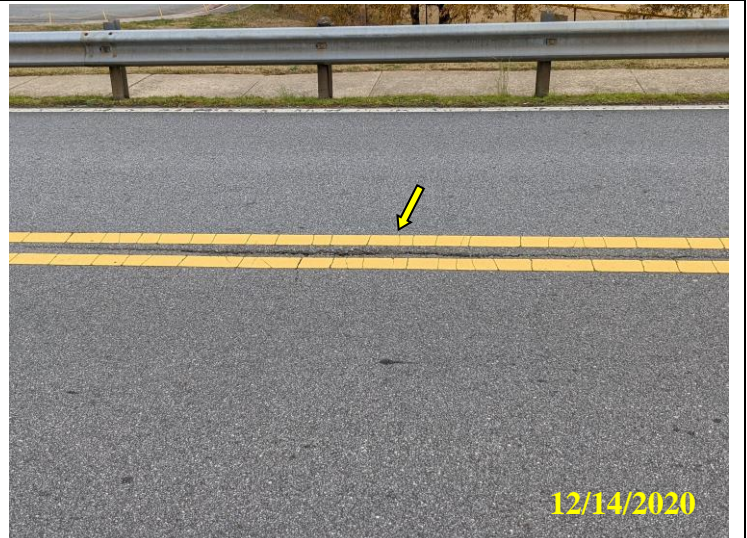
4. Additional crack in paved road on dam crest.
