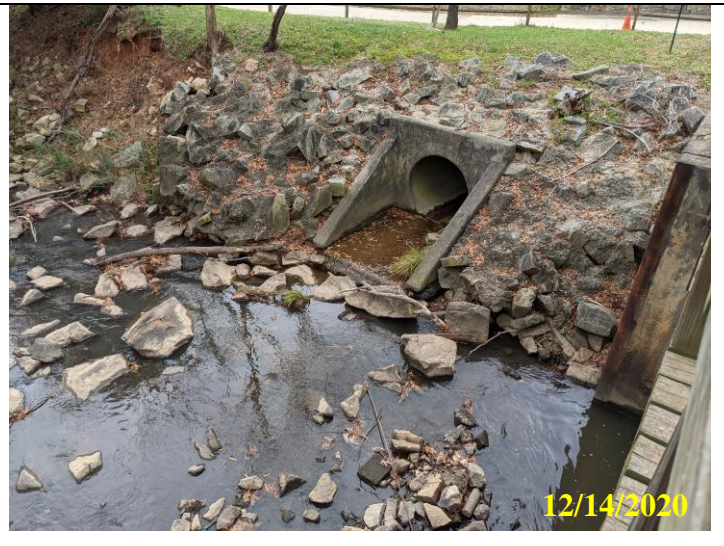
26. Erosion and undercutting observed near storm drain headwall downstream of plunge pool
