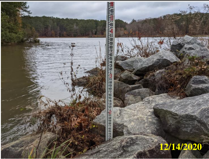
13. Inadequate riprap grading at the left wing wall of the concrete spillway resulting in erosion and undercutting of riprap
