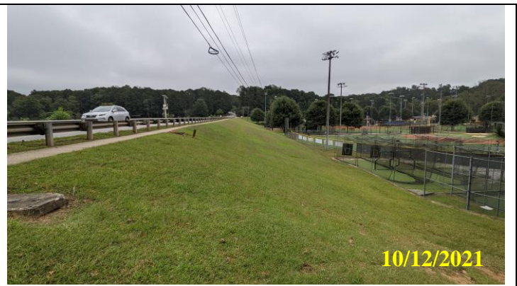
18. View of downstream slope looking toward left abutment
