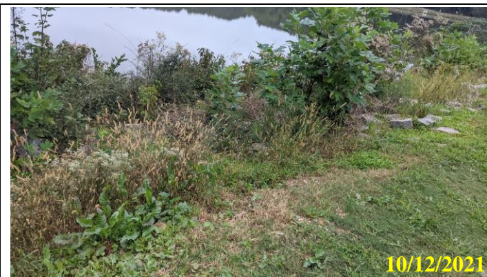
9. View of vegetation on upstream face of the dam
