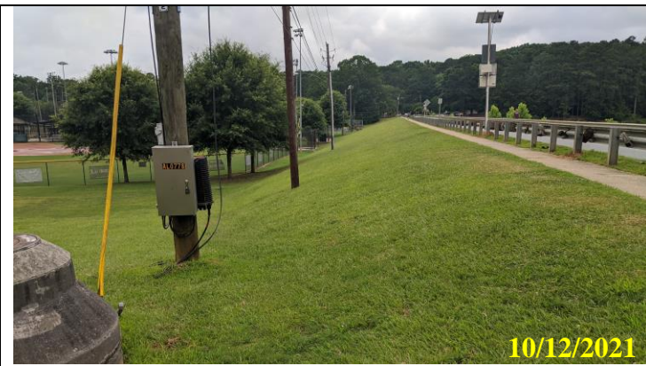
17. View of downstream slope looking toward right abutment
