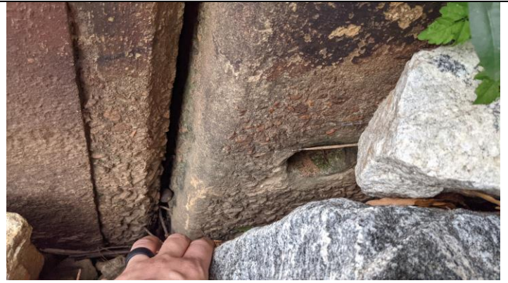
26. Matching toe drain on left side of plunge pool
