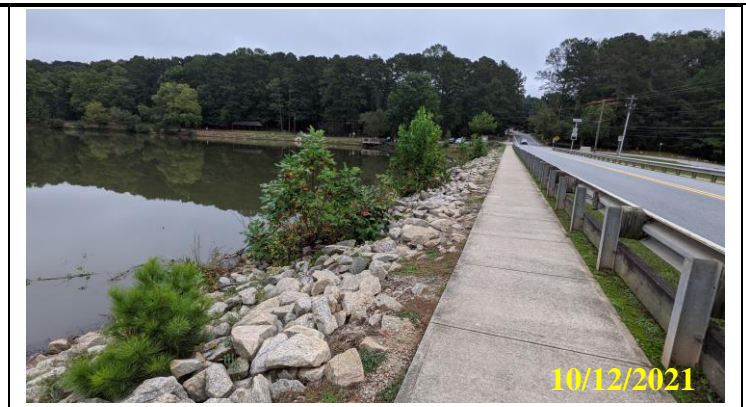
8. View of vegetation on upstream face of the dam
