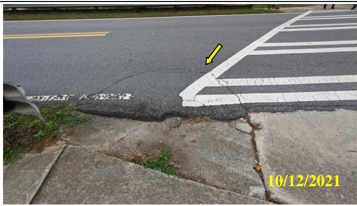
5. Depressed area on dam crest with crack on road pavement
