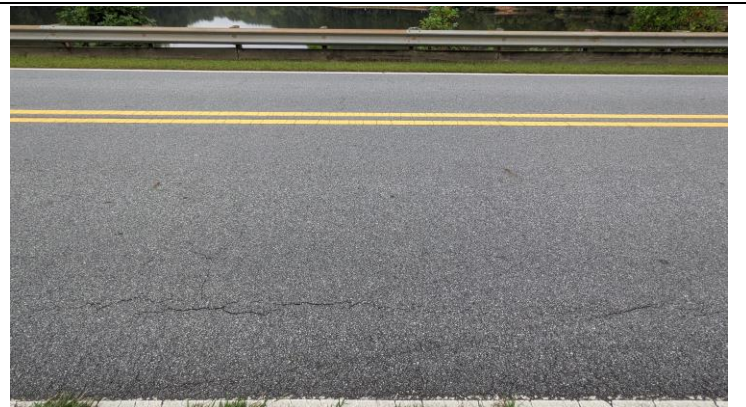
4. Additional crack in paved road on dam crest
