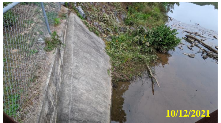
30. Vegetation and silt obstructing right side of upstream spillway. Sparse riprap along the right wing wall of the spillway
