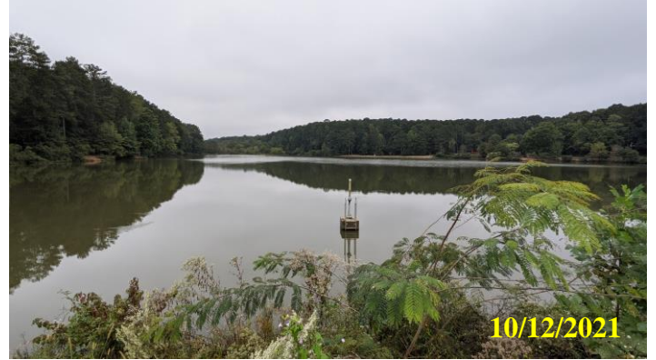
28. Principal spillway riser
