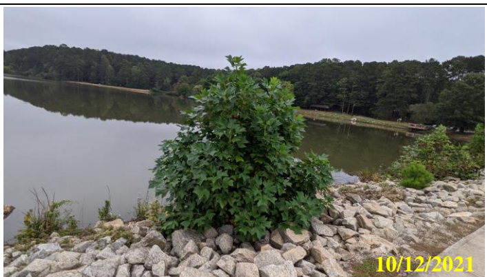
10. View of woody vegetation on upstream face of the dam
