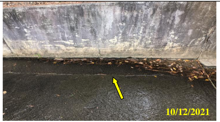
34. Previously completed repairs to spillway upholding well
