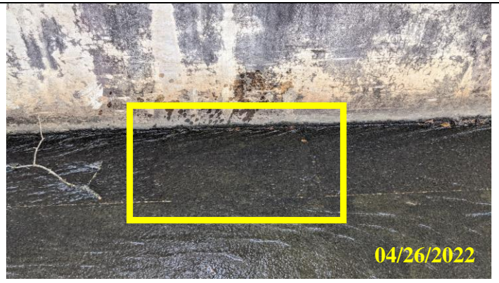
34. Previously completed repairs to spillway holding up well
