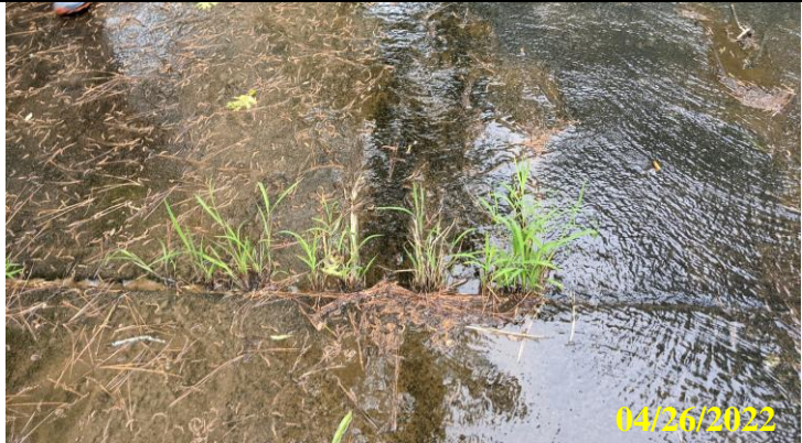
35. Grass growing between slabs in concrete spillway downstream of West Nancy Creek Drive
