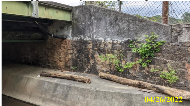
39. Vines and vegetation beginning to regrow on masonry wall downstream of bridge crossing
