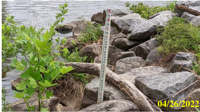
13. Inadequate riprap grading at the left wing wall of the concrete spillway resulting in erosion and undercutting of riprap
