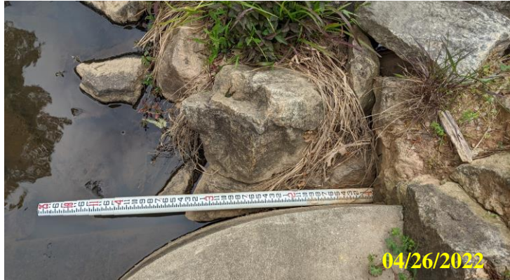
11. Inadequate riprap grading at the left wing wall of the concrete spillway resulting in erosion and undercutting of riprap. See Photo 12 for location of this photo.
