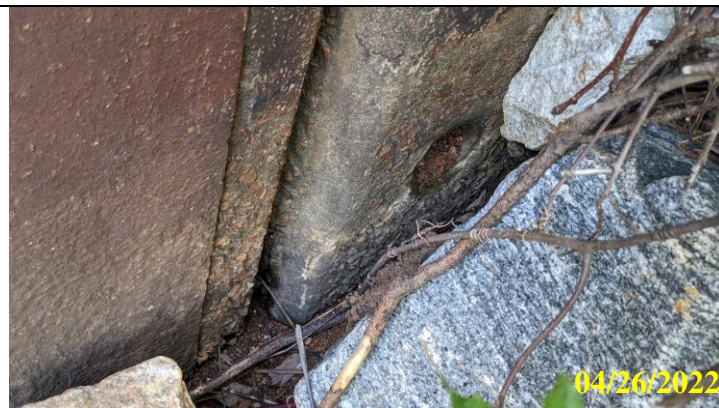
26. Matching toe drain on left side of plunge pool
