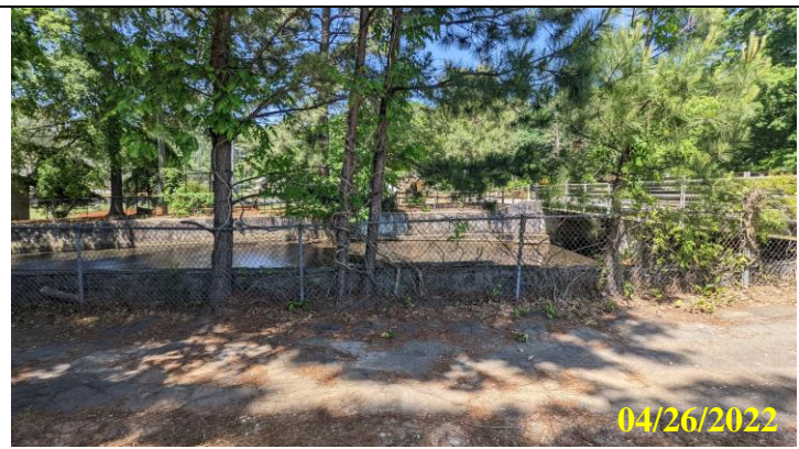
42. Trees at spillway fence, growing directly adjacent to and touching masonry wall
