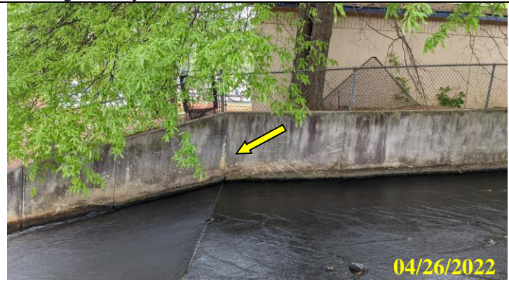
44. Cracked and missing concrete at top right of plunge pool face
