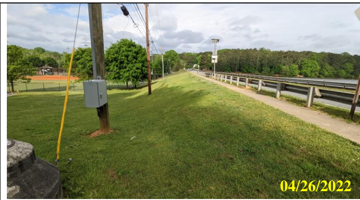
17. View of downstream slope looking toward right abutment
