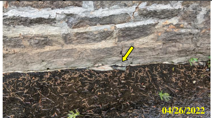
32. Concrete spillway cracking and uplift at masonry wall joint with exposed seal
