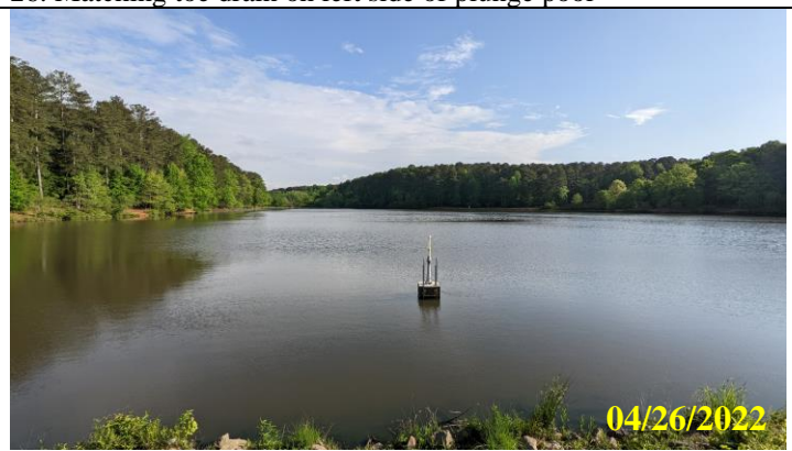
28. Principal spillway riser
