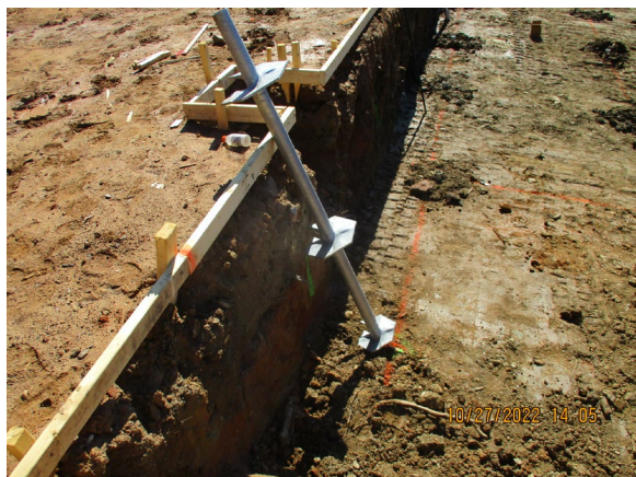
Helical piles installed under pool
