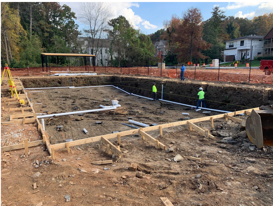
Excavated pool with plumbing install
