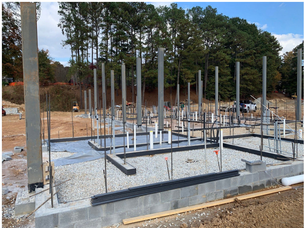
Helical piles installed under pool
