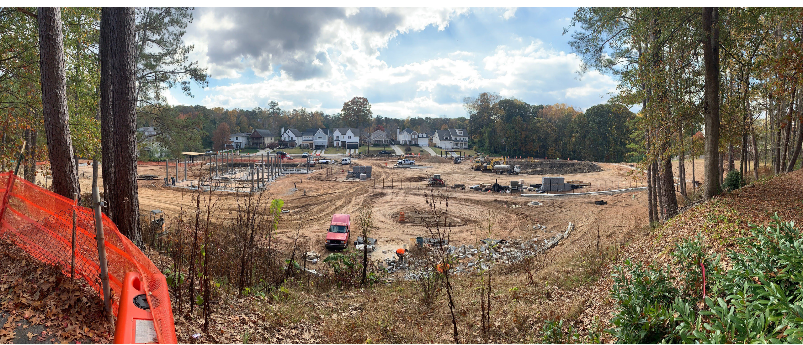
November 3, 2022, Panorama of Lynwood Park splashpad project: poolhouse steel columns on left, excavated lap pool beyond poolhouse, splashpad is behind trees on left, circular dropoff is in middle, turf field will be where stockpiled soil is, perimeter fence is installed, and underground detention is complete.
