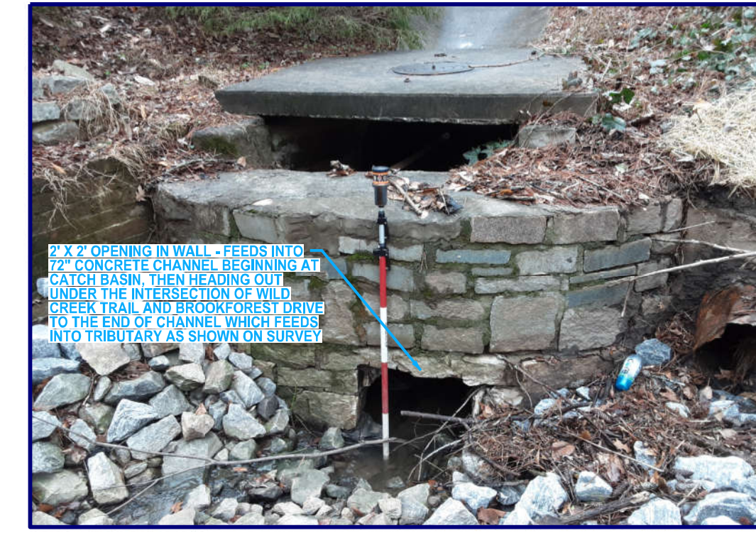
WALL STORM DRAINAGE IMAGE
