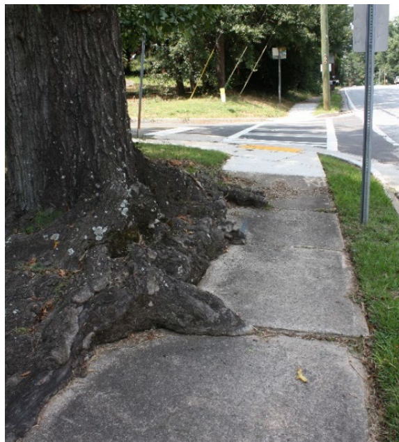
FIGURE 7. EXISTING SIDEWALK OBSTRUCTED BY TREE ROOTS NEAR CHILDERS ROAD OBSERVED DURING FIELD VISIT
