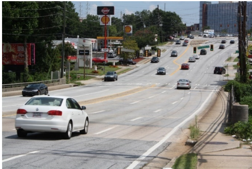
FIGURE 4. LOOKING SOUTH FROM BRIDGE OVER NORTH FORK PEACHTREE CREEK
