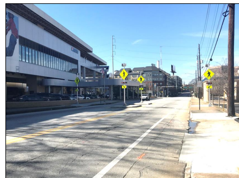
Rectangular Rapid-Flashing Beacon (RRFB) on Decatur Street in front of the King Memorial MARTA Station - pedestrian-actuated beacons alert motorists when people are crossing the road
