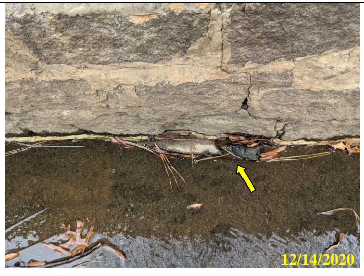
32. Concrete spillway cracking and uplift at masonry wall joint with exposed seal
