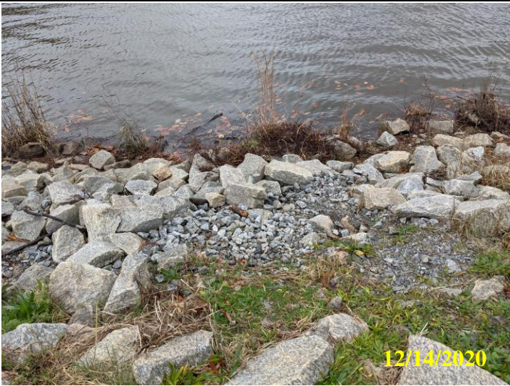
13. Inadequate riprap grading at the left wing wall of the concrete spillway resulting in erosion and undercutting of riprap
