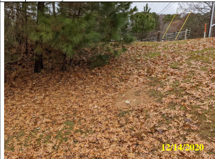
23. High traffic area at right side of downstream dam face showing erosion and missing grass
