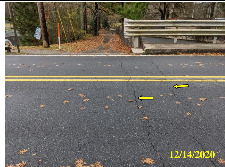
3. Cracks in paved road on dam crest at left bridge abutment.
