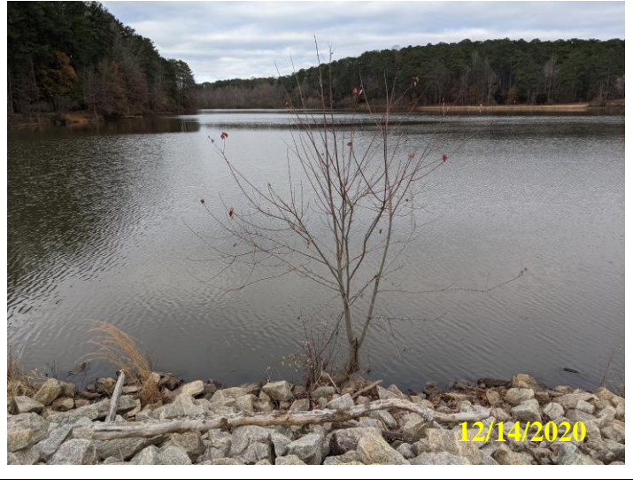
10. View of bare woody vegetation on upstream face of the dam
