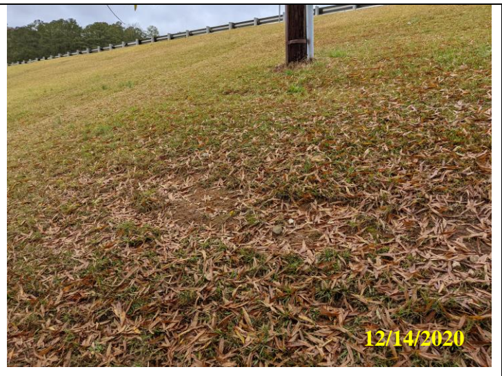
20. Patches of missing grass on downstream dam face
