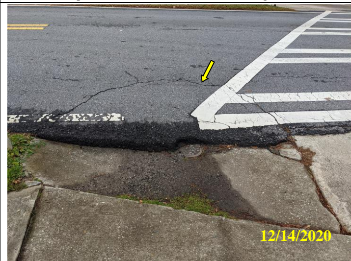
5. Depressed area on dam crest with crack on road pavement
