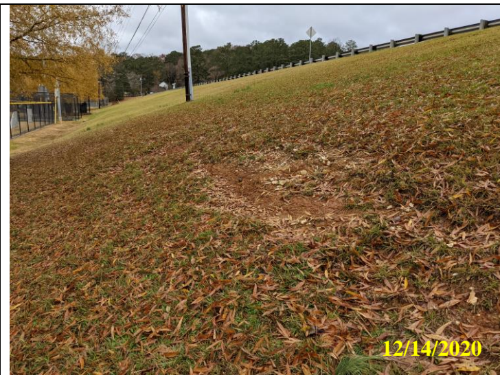
19. Patches of missing grass on downstream dam face
