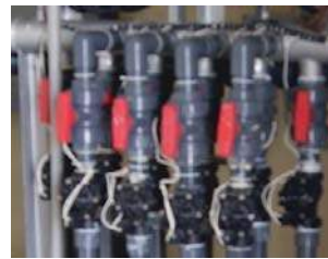
Manifold Housing and Water Hammer Arrester
