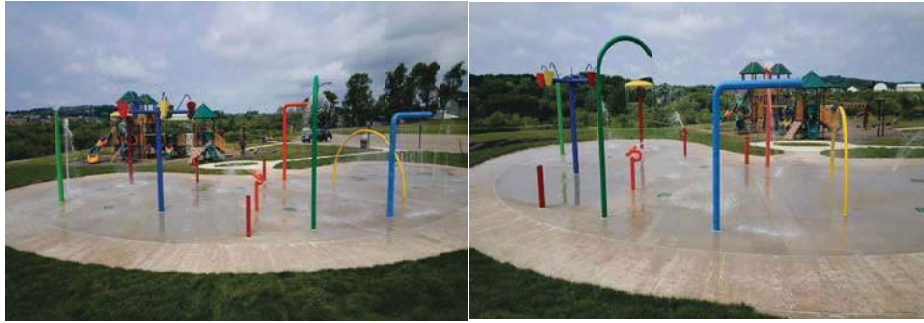
CHLOIE CREEK SPLASH PAD- ASBURY IA EQUIPMENT SUPPLY JULY 2017 2500 SQ FT Recirculation System w/ UV 23 Features Rod Schumacher, Project Manager rschumacher@conlonco.com 563.583.1724
