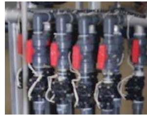
Manifold Housing and Water Hammer Arrester
