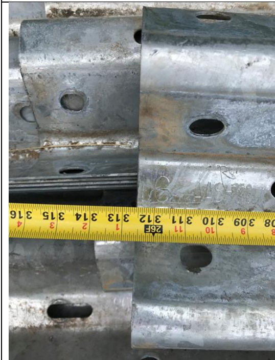
City furnished steel posts, w-beams, and spacer blocks to be installed in replaced section.
