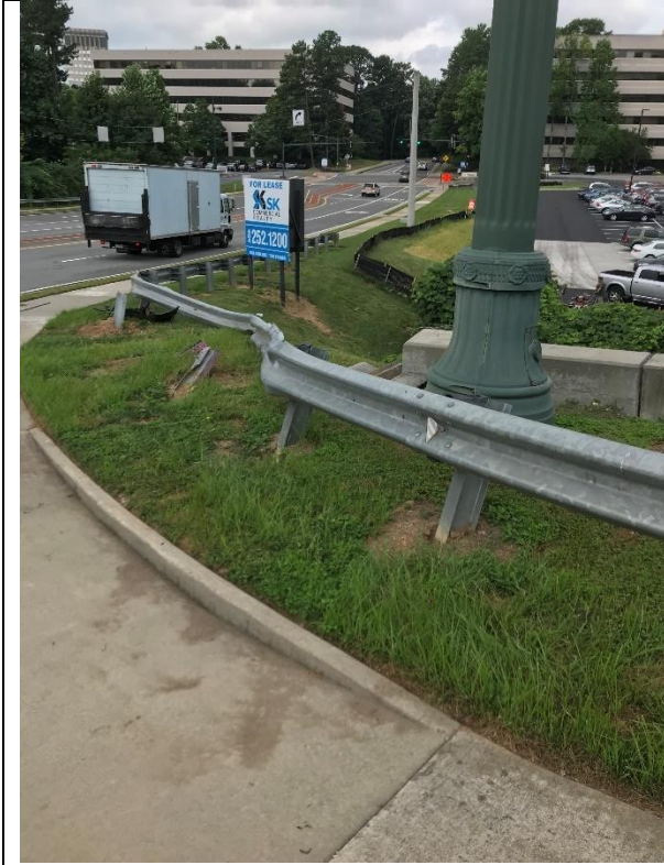
Photos of repair site and city furnished hardware
