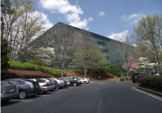
Large expanses of surface parking in this character area have the ability to accommodate additional development through the provision of structured parking decks.
