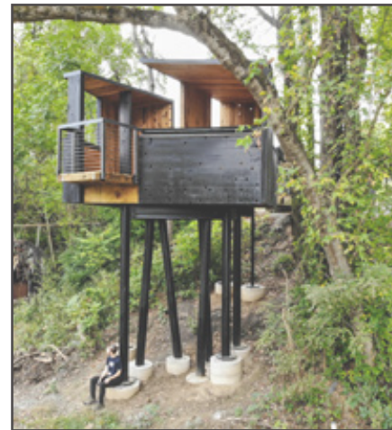
New River Train Observation Tower Radford, Virginia
