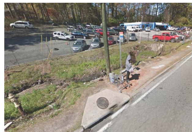
Examples of curb cut and sidewalk conditions on Buford Highway
