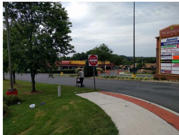
Existing sidewalk conditions at Northeast Plaza
