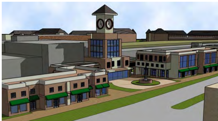
Brookhaven MARTA Station Redevelopment from Peachtree Road
