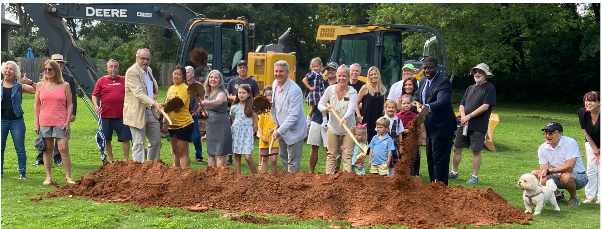
Brookhaven City officials, including District 3 Councilwoman Madeleine Simmons, Mayor Pro Tem Linley Jones, Mayor John Ernst, and District 4 Councilman John Funny, break ground on Langford Park improvements, which will include a new playground, Bocce Ball court, sheltered pavilion, and walking trails. The project should be complete by summer of 2023.
