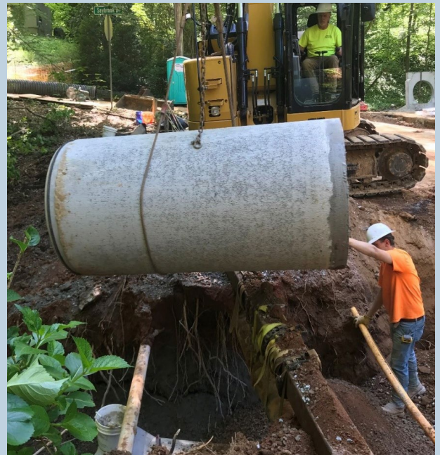
Above: Crews complete an overhaul of stormwater infrastructure at Inman Drive and Saybrook Drive in March 2020, replacing multiple smaller drainpipes with a single 36" culvert. Below: The stormwater issue before the upgrades.
