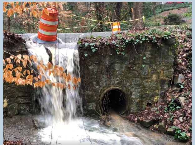
Above: Crews complete an overhaul of stormwater infrastructure at Inman Drive and Saybrook Drive in March 2020, replacing multiple smaller drainpipes with a single 36" culvert. Below: The stormwater issue before the upgrades.
