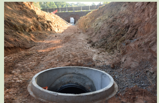
A new storm drain is part of the infrastructure improvements in Georgian Hills Park.
