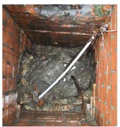
In places the corroded CMP is pitted/has holes in it. There is a belly in the downstream side of the pipe indicating subsidences or bedding/backfill erosion. The pipe should be replaced or lined. The upstream structure too should be replaced with standard GDOT structures, throats and tops.
