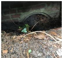
undersized and have no access for inspection or maintenance. The 18" culvert under Merriman is over ½ full with aggregate and other debris. The CB on the opposite side of the street is buried. The culvert at the west end of the street is buried and inspection / maintenance are not possible. Both sets of structures and pipe should be replaced with 18" RCP and median inlets.
